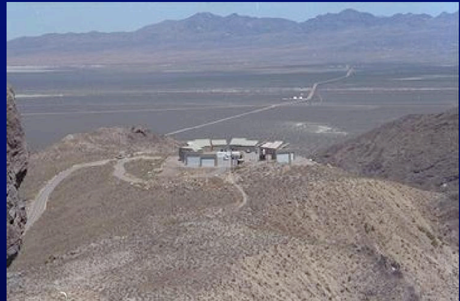
HiRes 2 on Camels' Back Dugway Proving Grounds, Utah
