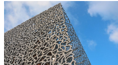
Museum of Civilizations in Europe and the Mediterranean (MuCEM) designed by Rudy Ricciotti: Ultra-High Performance Fiber-Reinforced concrete (UHPFRC)
