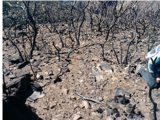
Sandstones: collapse of saturated colluvium on unrilled slopes and in gullies
